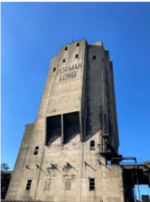
Figure 2.1 Current southern elevation.
