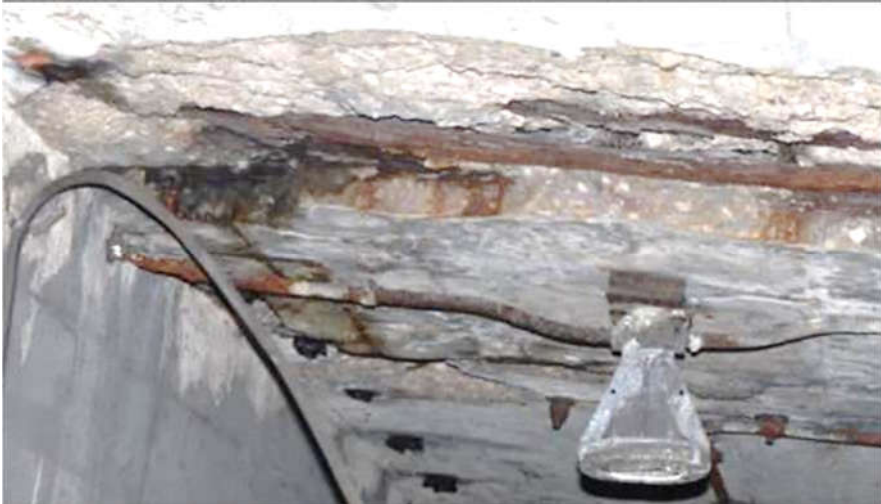
3 Internal Oven Cellar Roof
