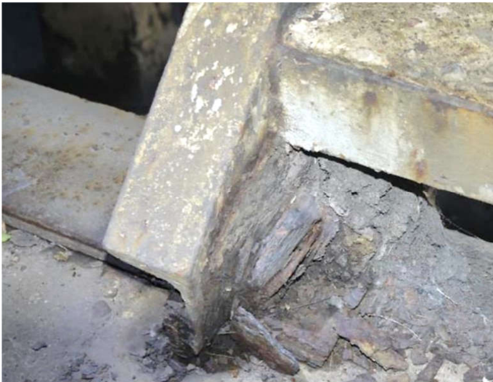
6 First Floor Stair Stringer Baseplate
