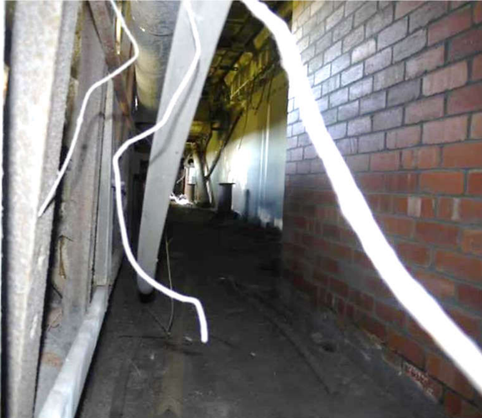
7 First Floor Corridor
