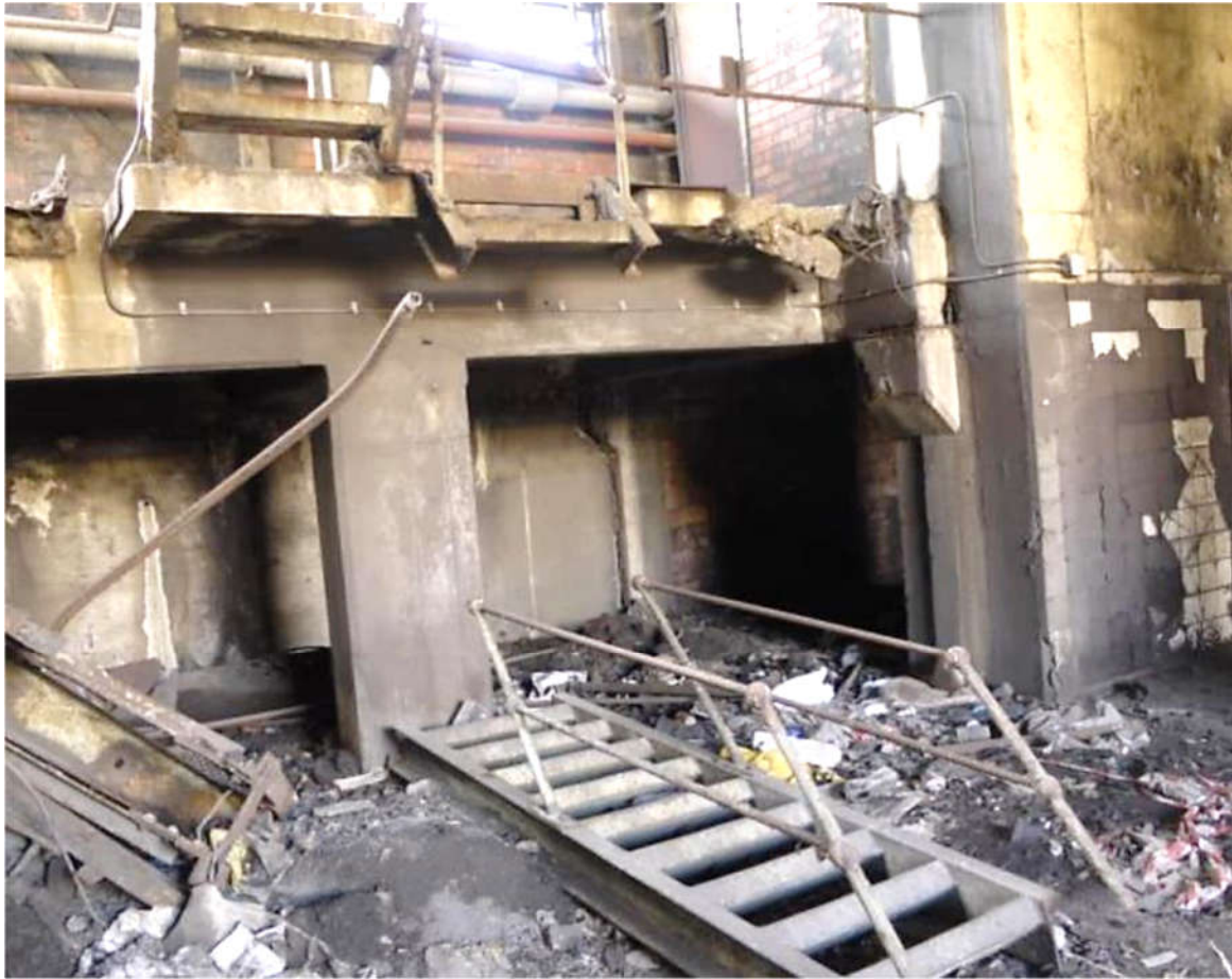
5 Internal Bunker Structure
