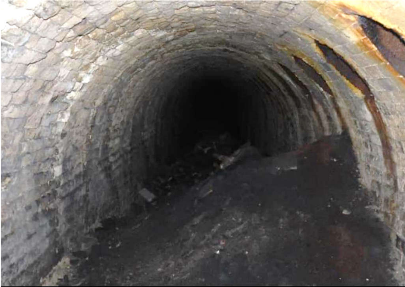
4 Chambers either side of Cellar
